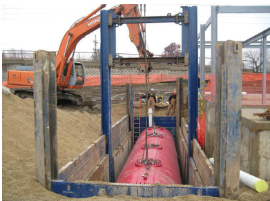
Slide Rail with Pit Configuration
