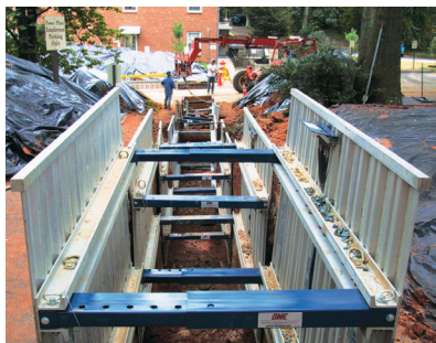
Hydraulic Aluminum Shield with End Loadable Struts
