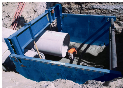
Height Adapter with Steel Trench Shield
