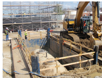
Clear Span Slide Rail with Tiebacks
